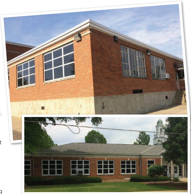
Top image: New windows on the left replaced the 57 year old originals, shown on the right. Bottom image: Pleasant Street Elementary School with window upgrade.
